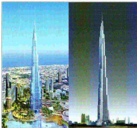
At a height of more than 700 m, the Burj Arab will be the highest building in the world and another milestone in the unprecedented construction boom which is taking place in the Emirate of Dubai
